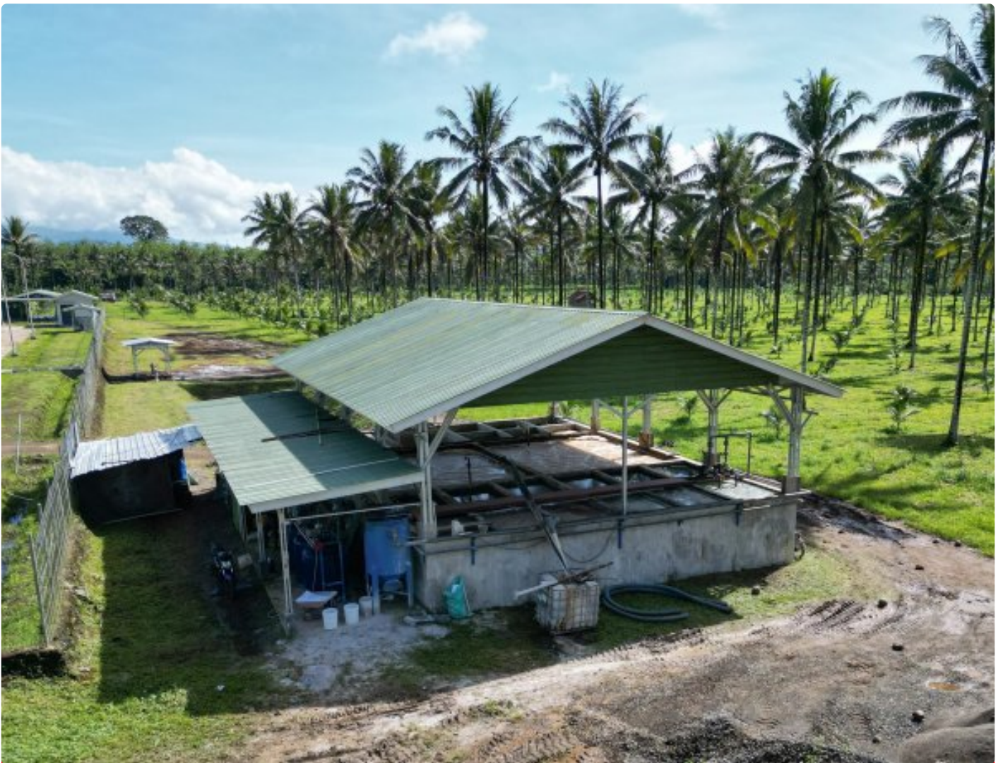
Dewacoco Waste Water Treatment Plant (WWTP)
